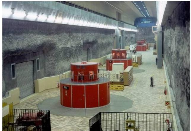
The lower reservoir, Kilburn Dam, is located in the foothills of the escarpment and has a capacity of 36 million cubic metres. The power station/pumping plant is situated more or less between the two reservoirs, 156 metres below the surface – equal to 52 storeys. The waterways connecting the two reservoirs are 2,9km long.
