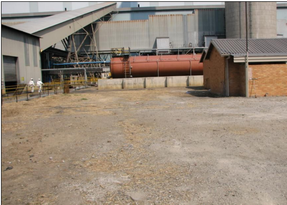
Figure 12: Current condition of positional Alternative 2
