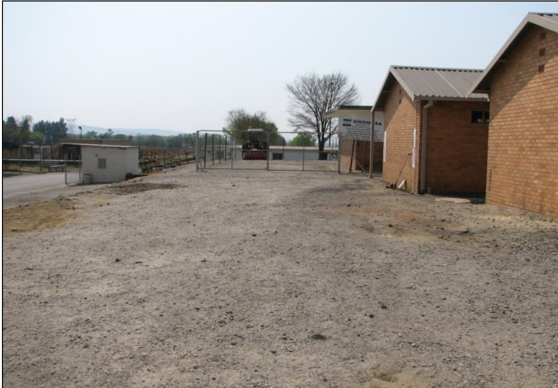
Figure 11: Current condition of positional Alternative 1
