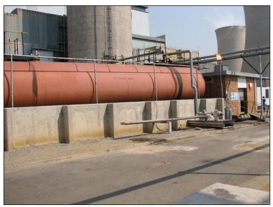
Figure 3: Photo of an existing fuel storage tank at the Grootvlei power station.
