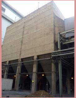
**Figure 2:** Existing Concrete ESP Casing within which the new Fabric Filter Plant will be installed, while extending the height of the casing with 1.1 meters.
