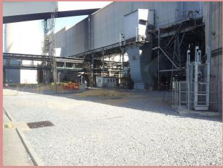
**Figure 3:** The area set aside for the construction of the proposed new compressor house (it is important to note that the entire area in the photo will not be utilised). This area was chosen due to its close proximity to the units.
