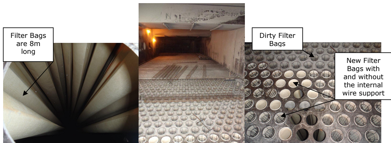
Figure 2: Inside a typical fabric filter plant
