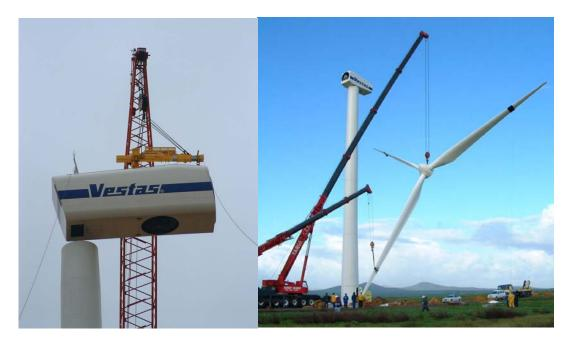
**Figure 7.6:** Photograph illustrating the assembly of a turbine (nacelle and blades) utilising a large lifting crane (photographs courtesy of Eskom from construction at the Klipheuwel demonstration facility)
