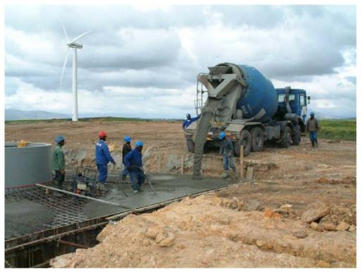
Figure 7.3: Photograph illustrating the construction of the foundation of one of the turbines at the Klipheuwel demonstration facility (photo courtesy of Eskom)
