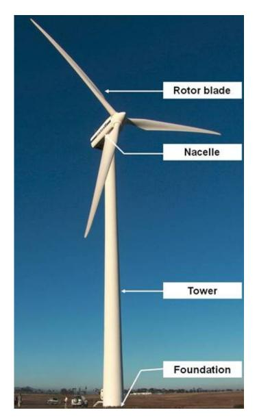
Figure 3.4: Illustration of the main components of a wind turbine
