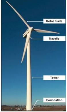
**Figure 1:** Illustration of the main components of a wind turbine<sup>1</sup>
