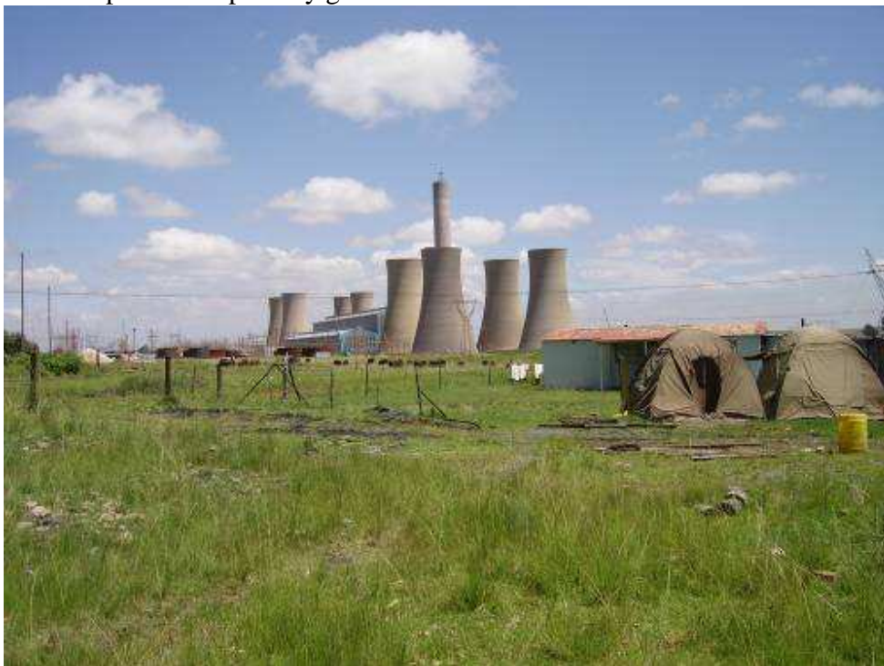
Plate 6: View along the powerline route from the R35 toward Komai Power Station. Note the residents and disturbance to the grass sward (dumping and overgrazing)
