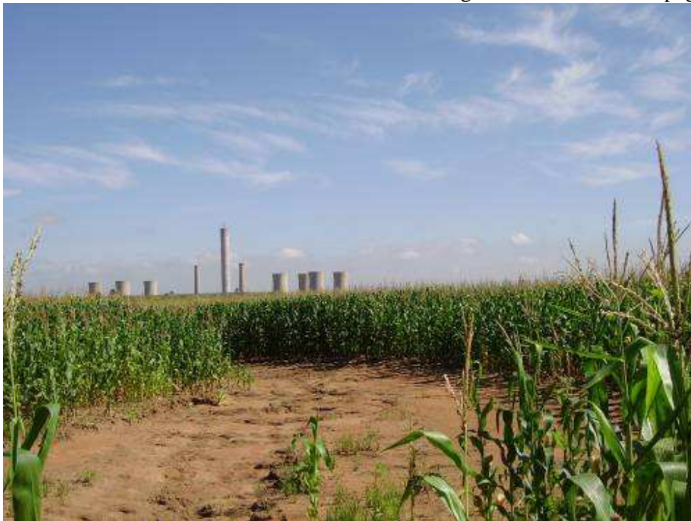
Plate 4: View of the powerline route in the maize fields at the southern end of the proposed deviation route.
