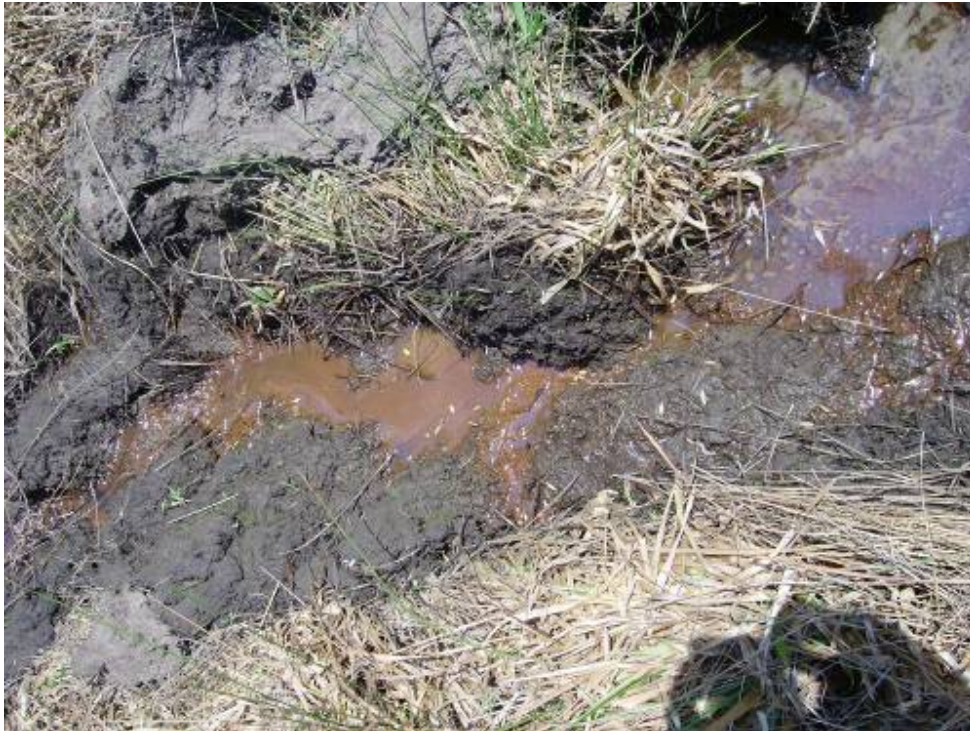
Plate 3: View of Ash dam Extension 3 Site showing extensive surface seepage.
