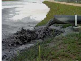
Ash slurry being pumped to the ash dam
