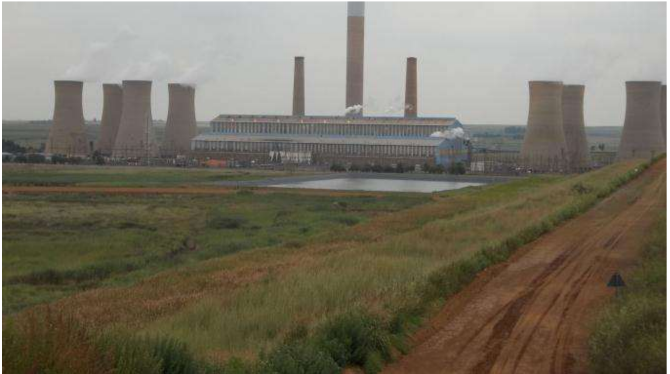
Plate 1: Current Status of Ash Dam Extension 3
