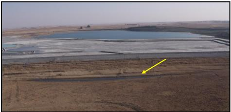
Figure 9-24 Drainage around the existing ash facility
