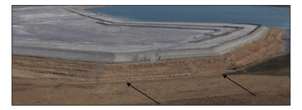
Figure 7-9: Rehabilitation on the existing ash disposal site in the foreground
