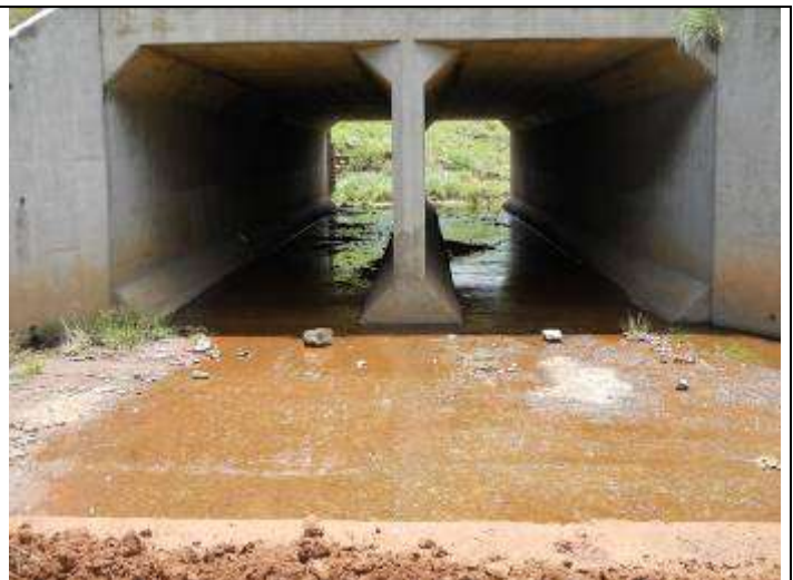
Figure 12: Downstream view of the CB5 site.
