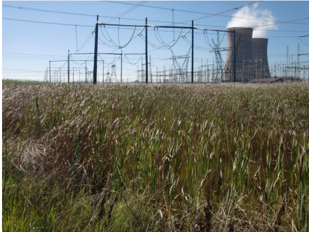
Photo 13. – Seepage at S03.
