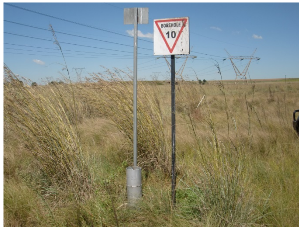
Photo 11. – Borehole B22 with wrong number plate.
