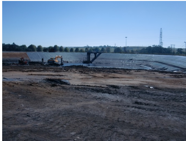
Photo 23. – Construction at coal stock yard dam P05.
