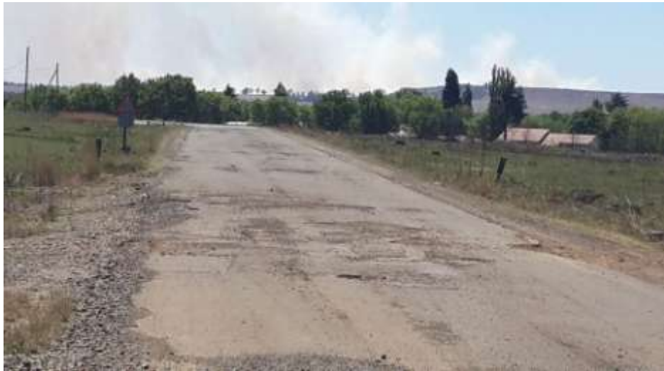
Road B from the Camden Village to the ash disposal facility
