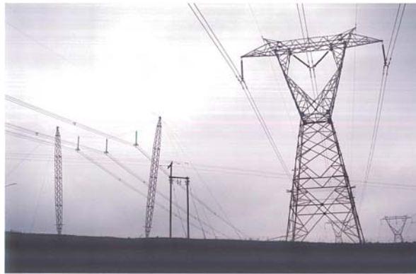
Plate 3.2.1.1 – 400kV Transmission Power Lines (Cross-rope Suspension & Strain Towers) crossing Distribution Power Line
