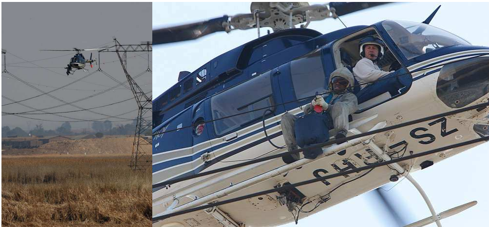
Figure 2: The installation of flappers on the shield wire from a helicopter.
