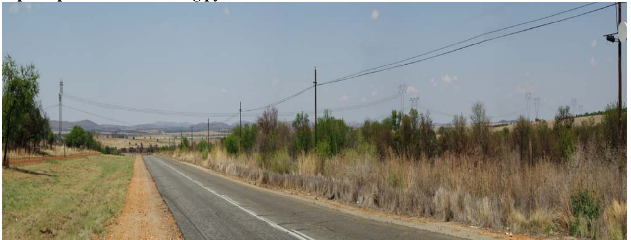
6-2 After: View of existing power line crossing Schoemansdrif Road with towers superimposed next to existing pylons.
