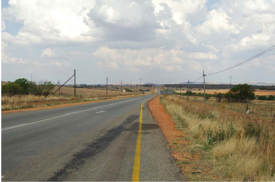
6-3: Before: Existing Power Line crossing R53
