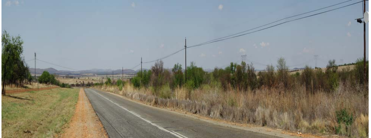
6-2 Before: Existing Line Crossing Schoemansdrift Road
