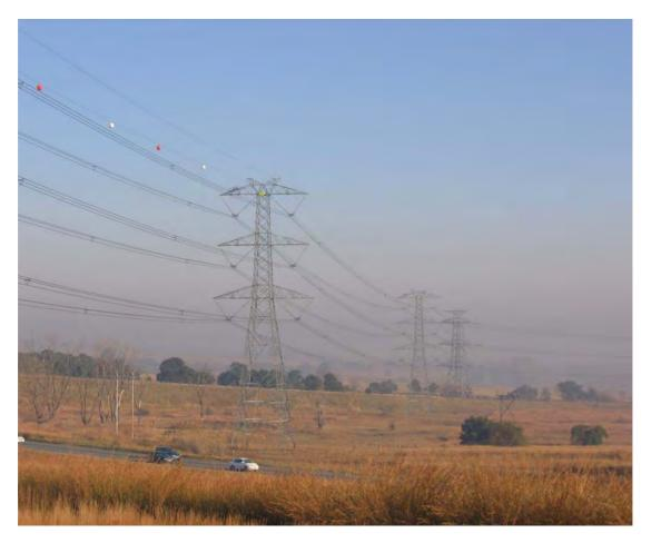
Figure 2.6: Self-supporting double-circuit tower
