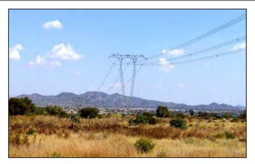
**Figure 2.7:** Guyed and Compact Cross-rope suspension tower typically used along the existing Dinaledi-Anderson 400kV transmission power line route
