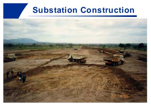
Photograph 2.1: showing earthworks for a substation site
