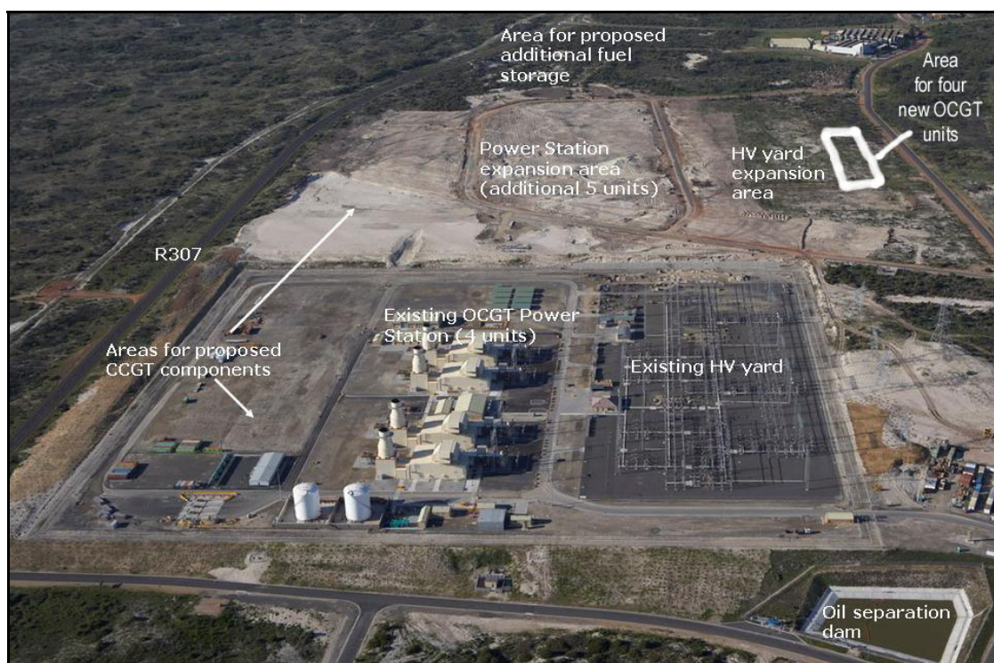
Figure 1: Aerial view of the Ankerlig OCGT power station (four OCGT units and two fuel tanks are shown).
