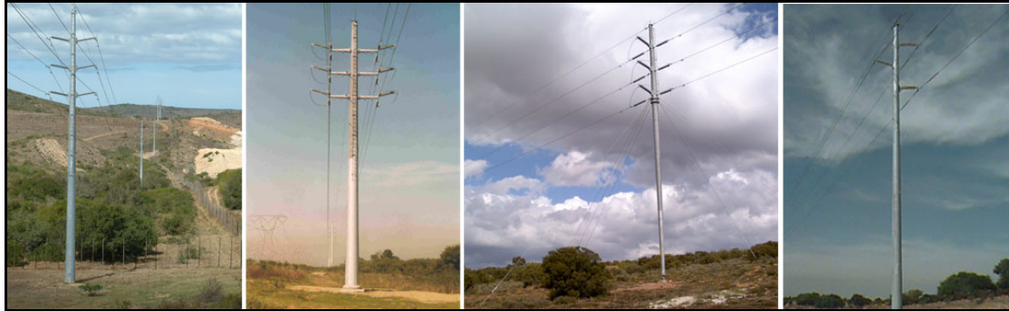
Figure 5: Examples of 132kV power line towers.
