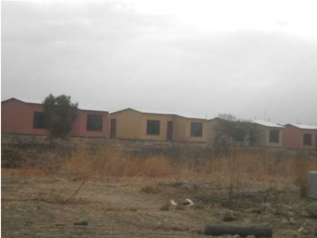
Figure 16: Google Earth image of the new housing developments in Mothulung
