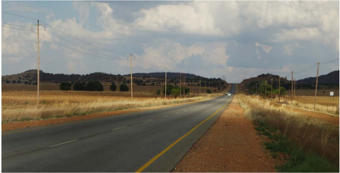
6-6: Before: Looking east along R53
