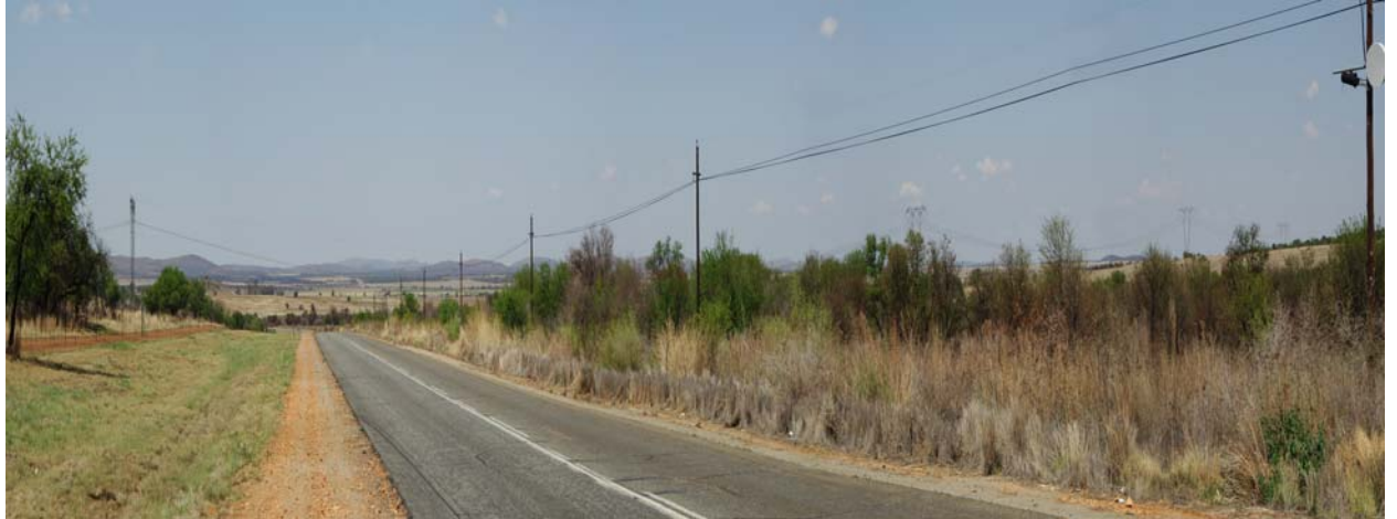
6-2 Before: Existing Line Crossing Schoemansdrift Road
