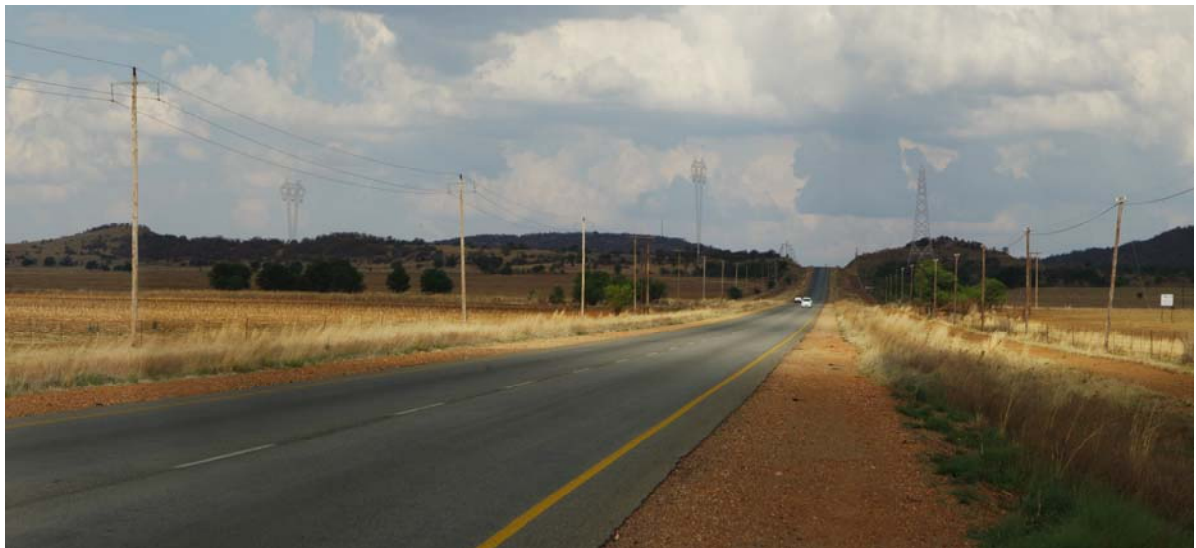
6-6: After: Looking east along R53 with towers indicating Western Alignment 1
