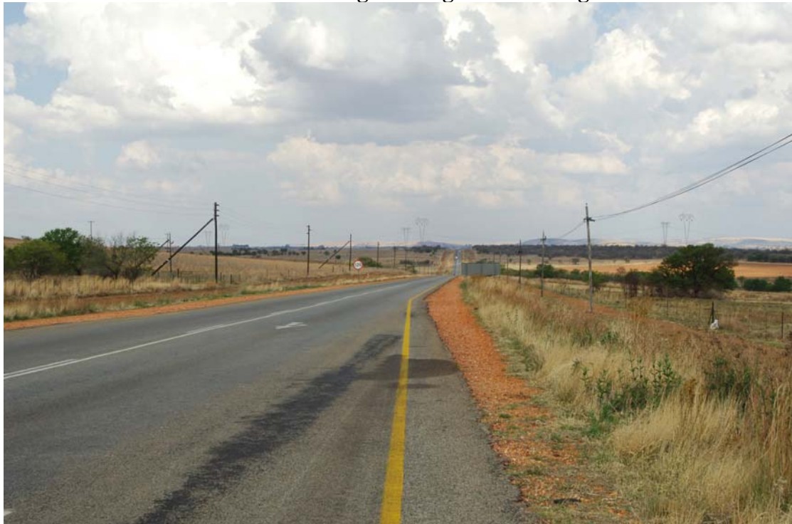
6-3: After: New Power Line following Existing Line crossing R53
