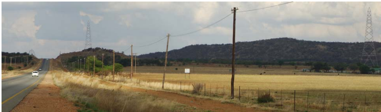
6-7: After: Looking south east along R53 with towers showing Western Alignment 1 alignment
