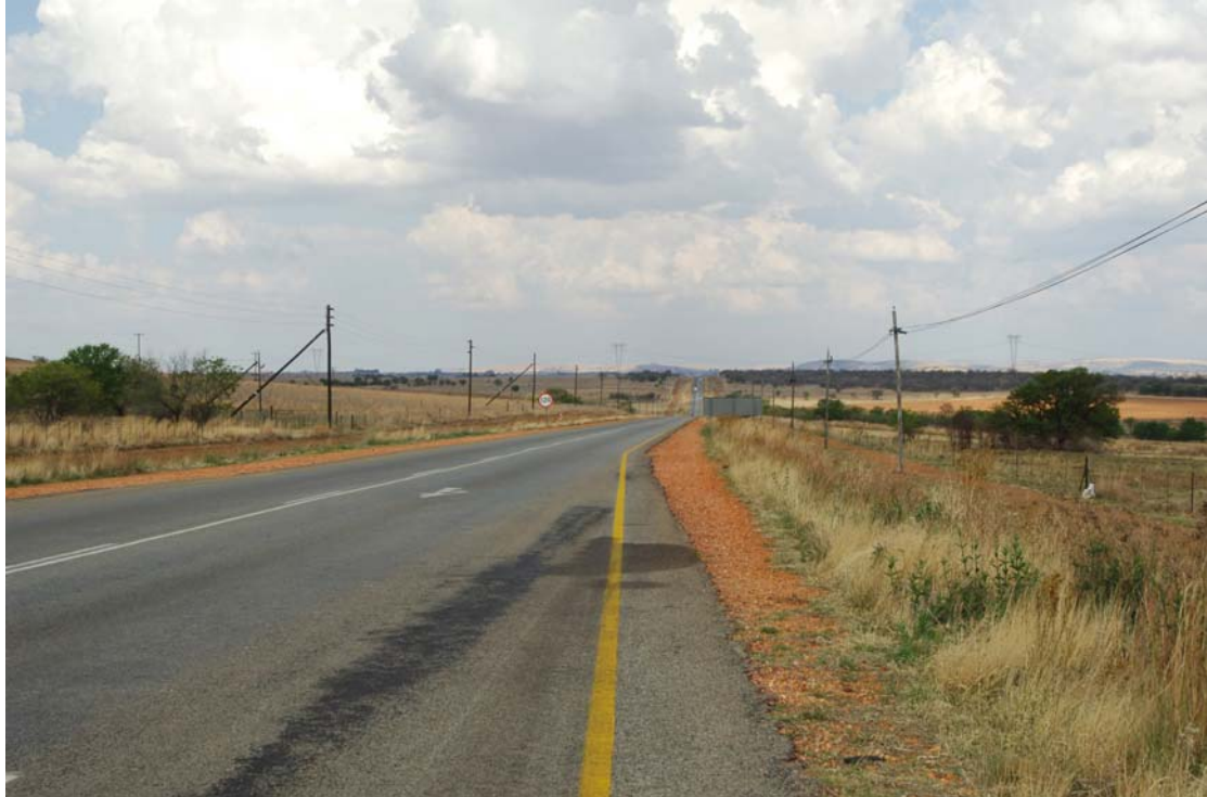
6-3: Before: Existing Power Line crossing R53
