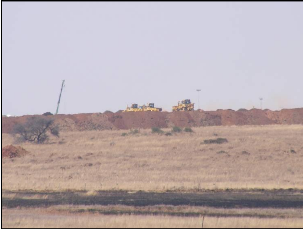
Figure 4-2: Current construction activities on site
