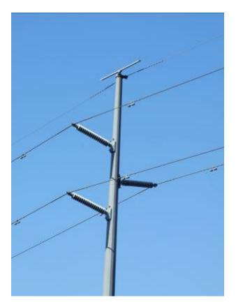
Figure 4: Single steel pole 88/132kV sub-transmission structure
