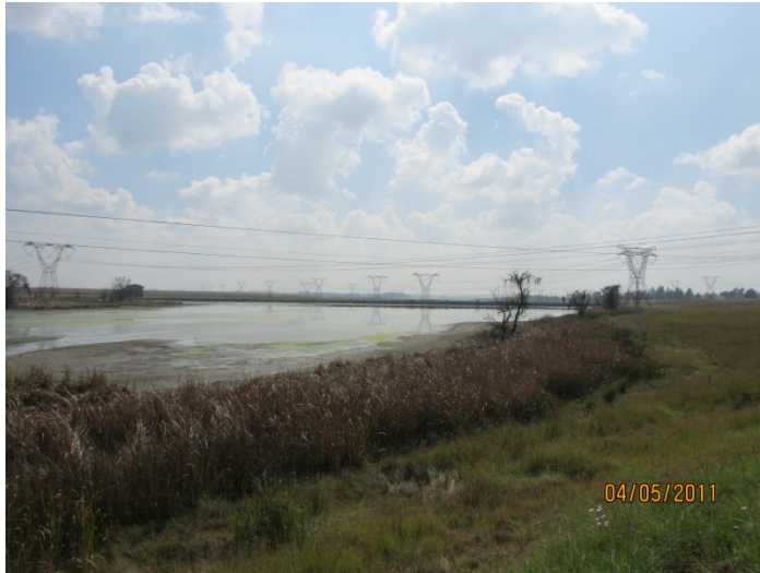
Figure 6: A dam observed close to Alternative B.
