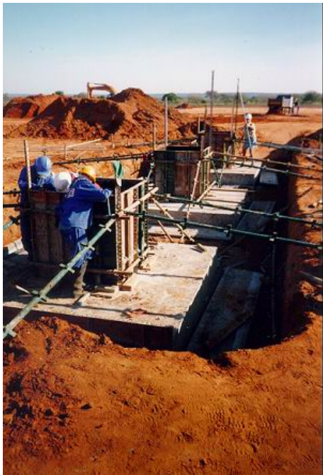
PHOTOGRAPHS 6 AND 7: TRANSFORMER FOUNDATIONS
