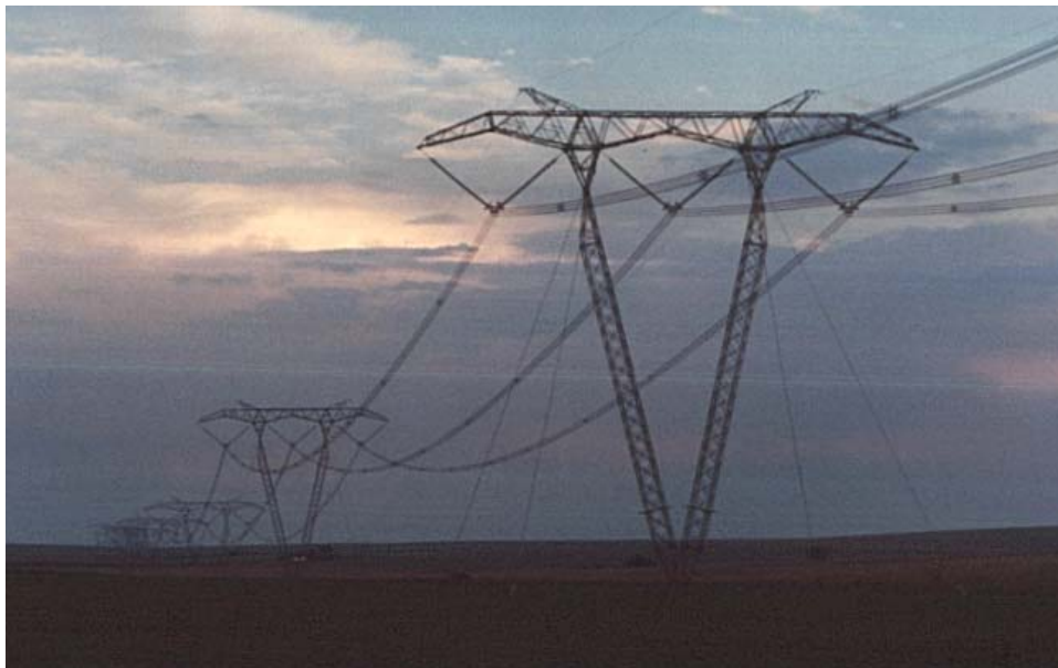
Figure 3: Example of Guyed V Tower Structure
