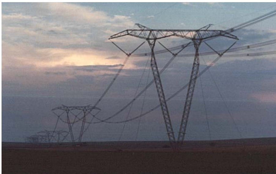
Figure 2: Example of Guyed V Tower Structure
