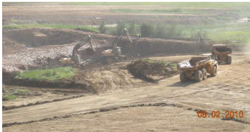
Example of Construction at Kusile Power Station
