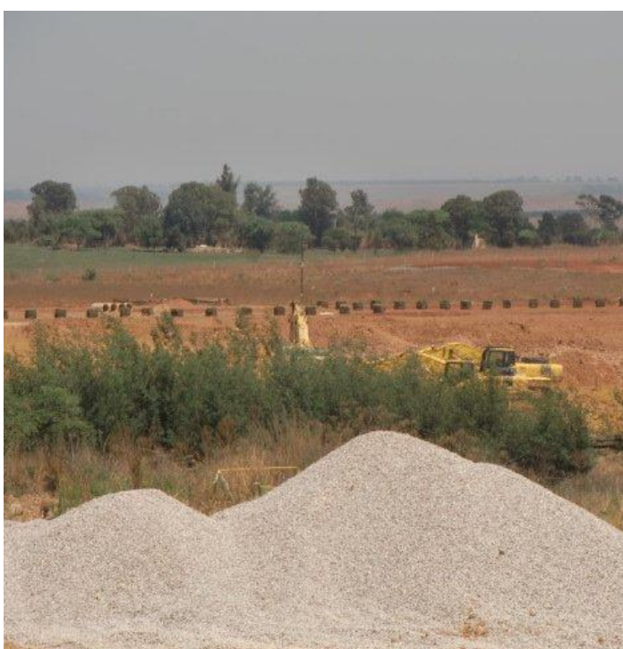
Construction at Kusile Power Station
