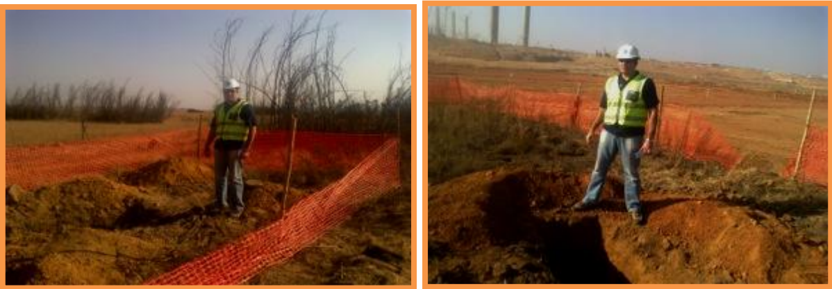
Plates 12 and 13: View of Eskom supervisor inspecting excavated pits.
