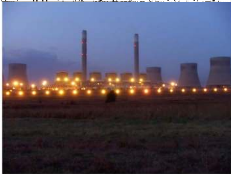
VIEW OF POWER STATION AT DUSK FROM 1.7 KM
