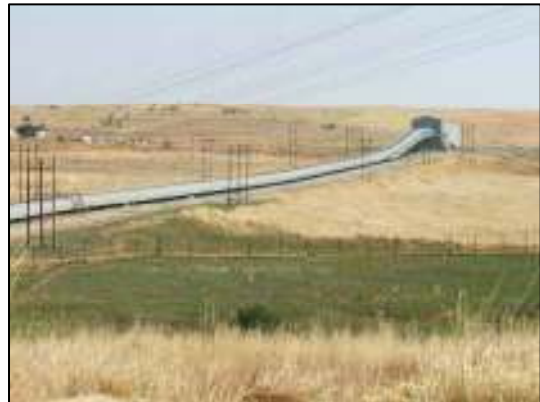
Figure 5: Typical conveyor system
