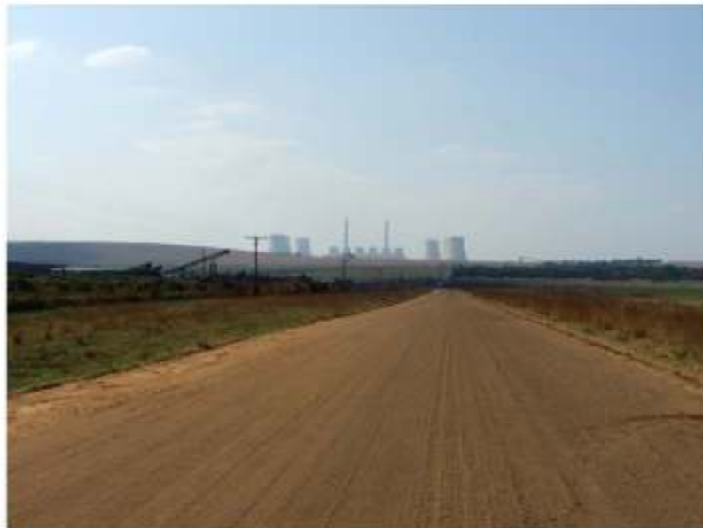
VIEW OF POWER STATION DURING DAY TIME FROM 5KM
