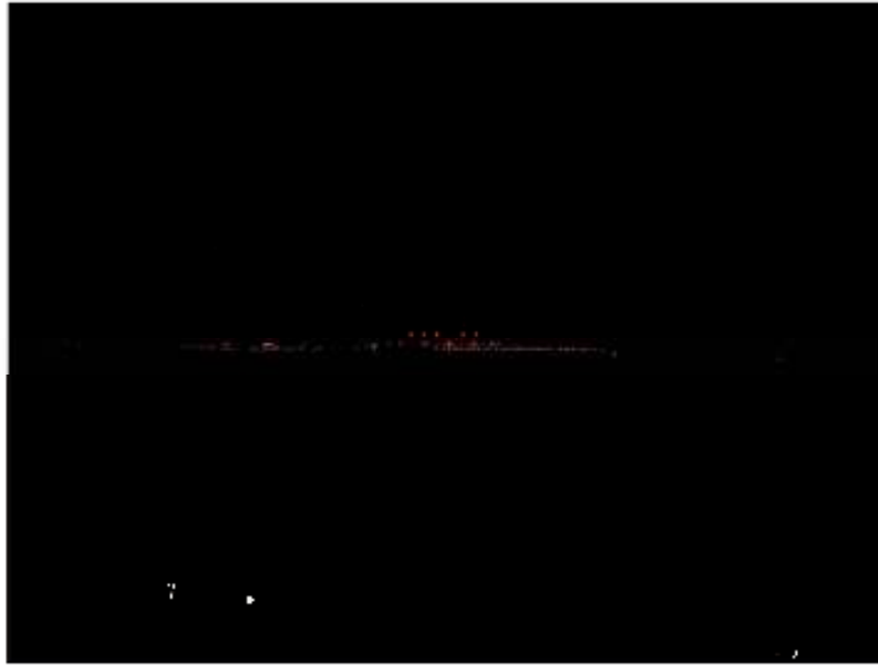
VIEW OF POWER STATION AT NIGHT FROM 6.3 KM
