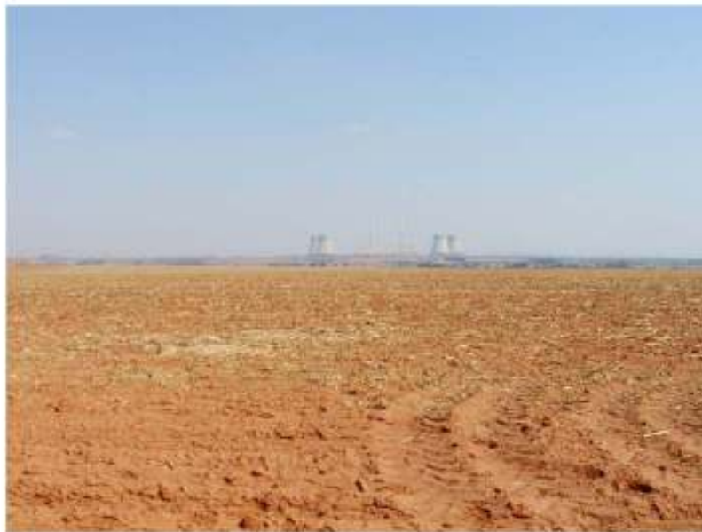
VIEW OF POWER STATION DURING DAY TIME FROM 6.3 KM
