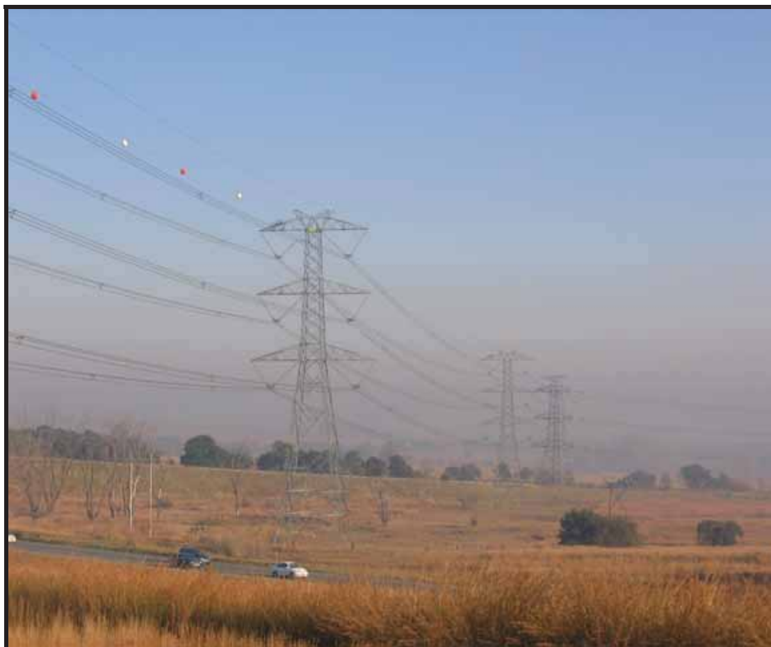
Figure 2.13: Self-supporting double-circuit tower
