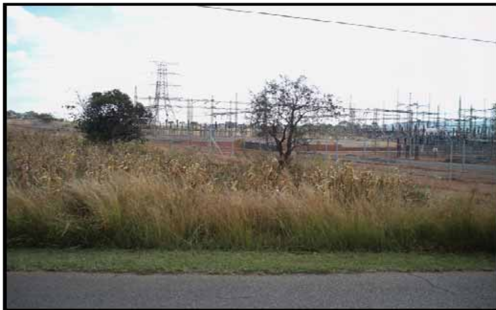
Figure 2.5: View of the existing Kwagga substation when viewed southwards from Church Street
