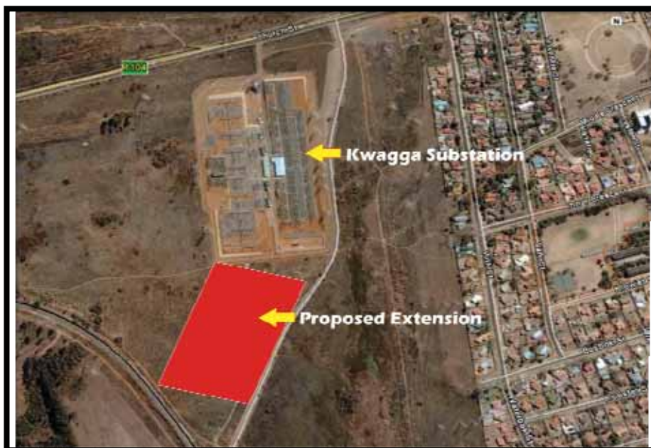
Figure 2.6: An aerial view of the existing Kwagga substation and the proposed extension to the substation site
