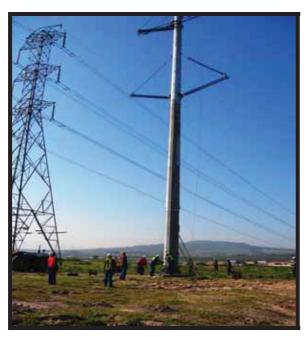
**Figure 6.6:** Example of a self-supporting double circuit tower and a monopole tower that can be used where there are space constraints.
