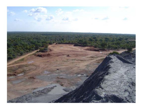
Figure 11.10: Cleared area for the expansion of the existing Matimba ash dump.
