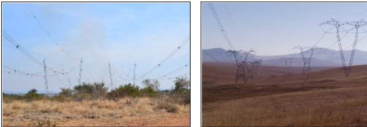
Figure 8: Difference between cross rope suspension towers (left photo) and self support towers (left in right photo) and a guyed suspension tower (right in right photo)
