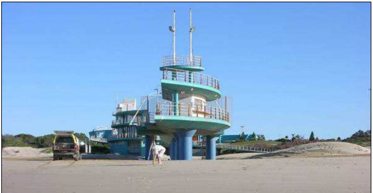
Figure 4.3. An example of a "bridge" shaped so that airflow under the bridge is accelerated, so there is no build-up of sand under the bridge. The dominant wind blows from left to right. A small dune forms at times upwind of the bridge (left), and a large dune forms downwind of the bridge (right).
