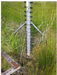
This type of electrified fence is an unmitigated disaster! Note the small gaps between strands and the many electrified strands near ground level.
