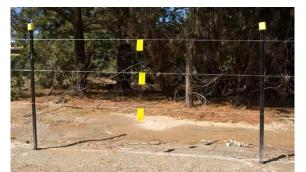
Visibility of fencing can be improved using either plastic or aluminium tags or other types of flagging. Flags should be spaced no wider than 30cm. Note that if you use plastic
