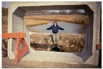
www.massaudubon.org/.../ restoration.html This restrictive culvert at Argilla Rd. in Ipswich has now been replaced by a much bigger box culvert, allowing the natural flow of the tide.
