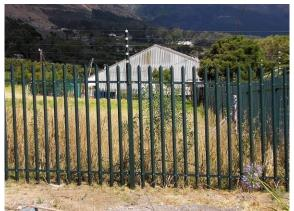
The palisade fence is OK, but the electrified wires at the top are not visible enough and therefore pose a threat to birds.
