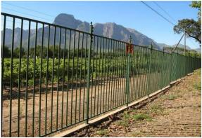
This palisade fence would be good if the concrete wall at the bottom were flush with the ground.
