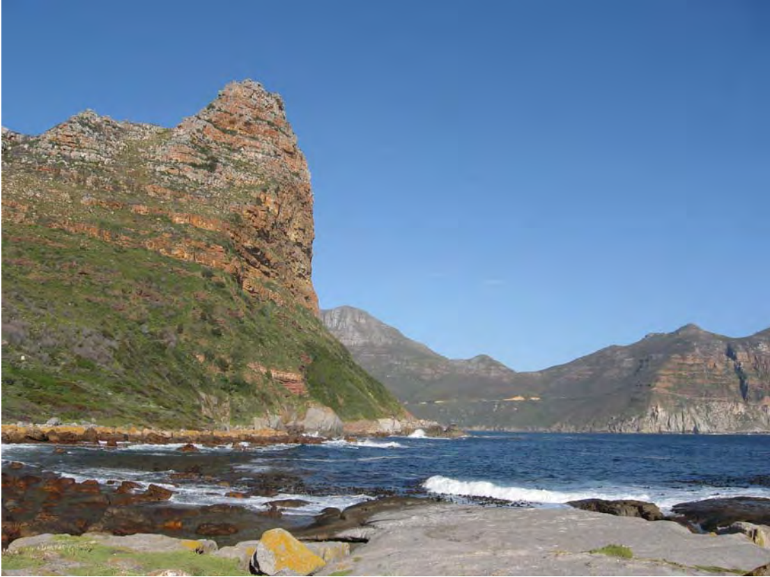
Figure 10. Precipitous cliffs comprising highly fractured and jointed Palaeozoic quartzites at the entrance to Hout Bay, posing a threat of tsunamigenic rockfalls to the town itself, with some dwellings and infrastructure at only 1.5 m asl.
