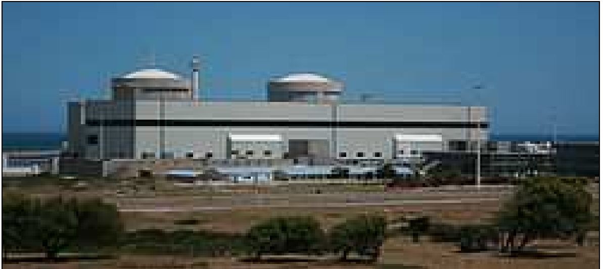
Figure 3.2: Koeberg Nuclear Power Station
