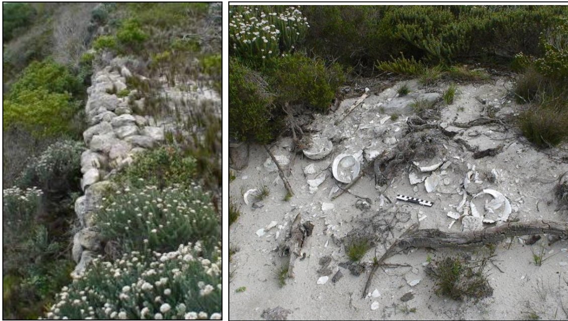
Figure 8 (above left) Historic limestone boundary wall, Bantamsklip.
