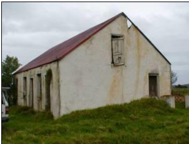
Figure 19 (below left) This cottage close to Welgelegen is the only generally protected building in the study area
