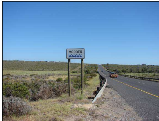
Figure 7.18: Modder River Bridge along the R27
