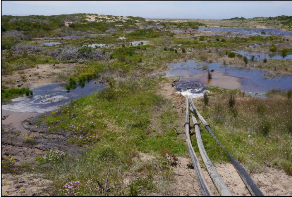
Figure 8.2 Above: An interdune pond in the Santareme dunefield “upstream” of the pond that ruptured on 15 September 2012. Left: three pipes were installed as siphons to drain the pond gradually, so as to avoid a further flashflood.
