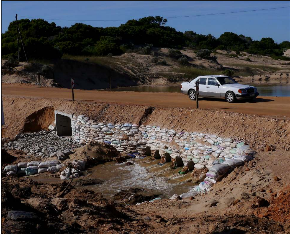
Figure 8.4 The temporary culvert over the Sand River built in October 2012
