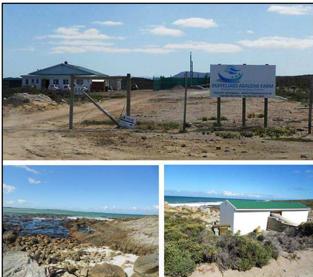
Figure 4-20: Bantamsklip – Buffeljags abalone farm and seawater intake area with pump station
