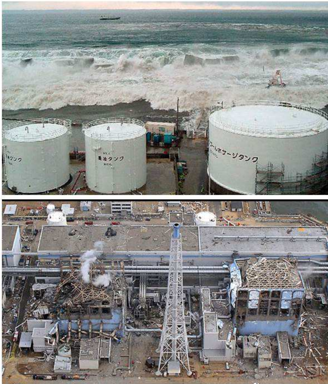
Figure 2-7: Tsunami waves approaching the Fukushima Dai-ichi NPP (top) and a view of the damaged reactors 3 and 4 (bottom)
