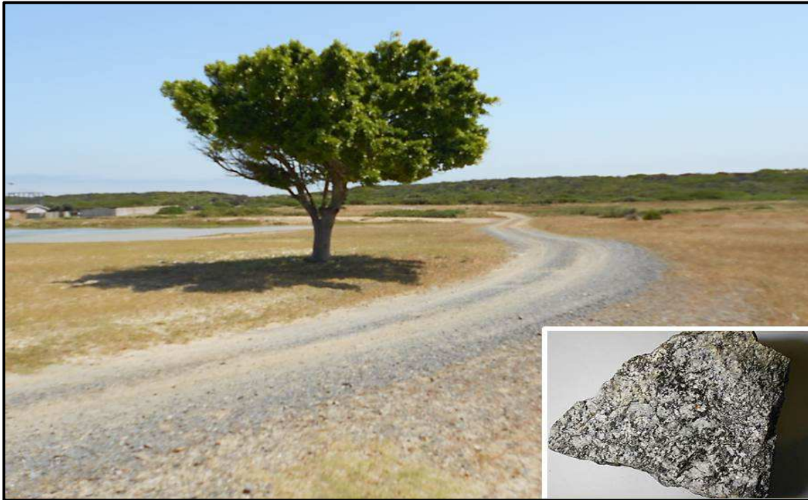
Figure 4-31: Aggregate used for dirt road construction on the dune surfaces of the Duynefontein site
