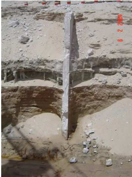
Figure 1: Example of cut-off wall used at Coega Harbour
