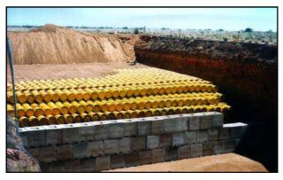
Figure 3-16: Low Level (steel) and Intermediate Level (concrete) radioactive waste drums (respectively above and below) at Vaalputs. The drums are covered with layers of clay.
