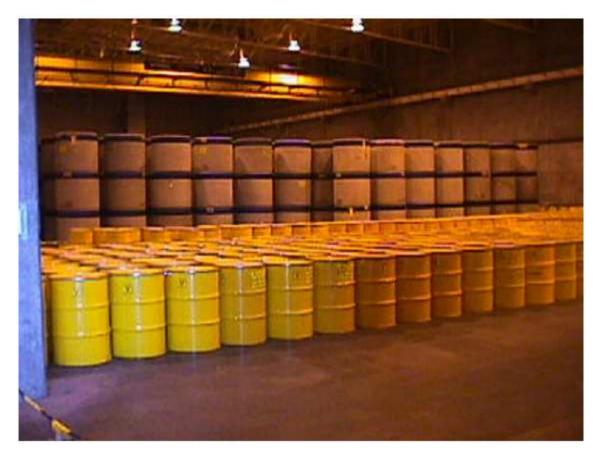
Figure 3-14: Storage facility for ILW and LLW showing concrete drums in the background and steel drums in the foreground
