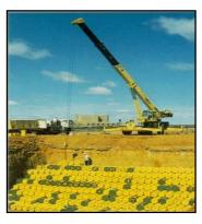
Figure 3-17: Placement of Low Level Waste steel drums at Vaalputs
