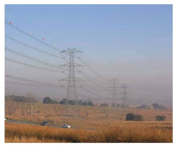
Figure 2.6: Self-supporting double-circuit tower
