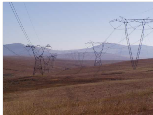
Figure 6: Difference between cross rope suspension towers (left photo) and self support towers (left in right photo) and a guyed suspension tower (right in right photo)
