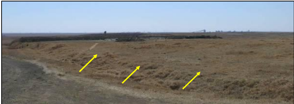
Figure 4-3: Existing waste disposal site with capped and rehabilitated area in the foreground
