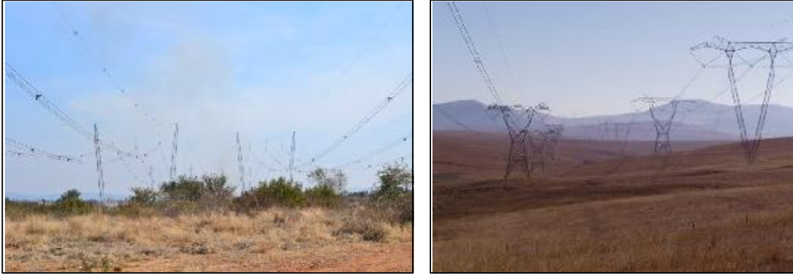
Figure 18 - Difference between cross rope suspension towers (left photo) and self support towers (left in right photo) and a guyed suspension tower (right in right photo)
