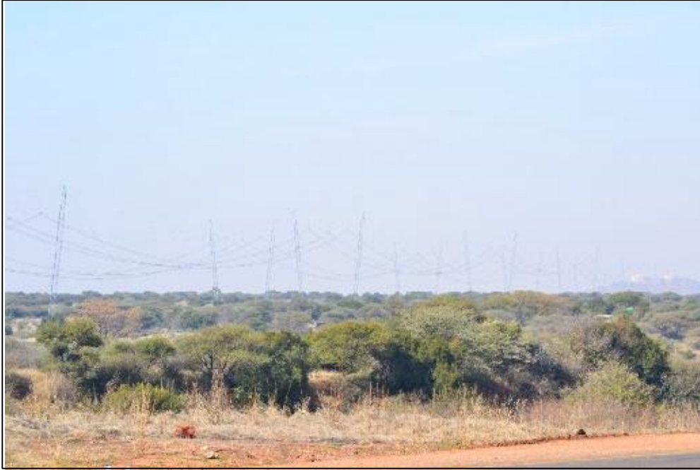
Figure 13 – An example of 2 parallel lines with cross rope suspension towers in the Sun City Area of the North west Province
