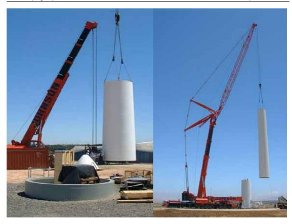
Figure 7.6: Photograph illustrating the assembly of a turbine tower utilising a large lifting crane (photographs courtesy of Eskom taken during the construction of the Klipheuwel demonstration facility)
