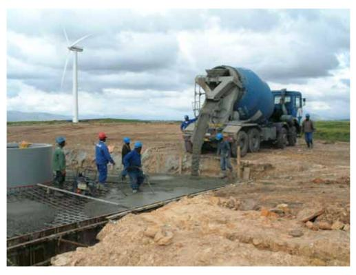
**Figure 7.4:** Photograph illustrating the construction of the foundation of one of the turbines at the Klipheuwel demonstration facility (photo courtesy of Eskom)
