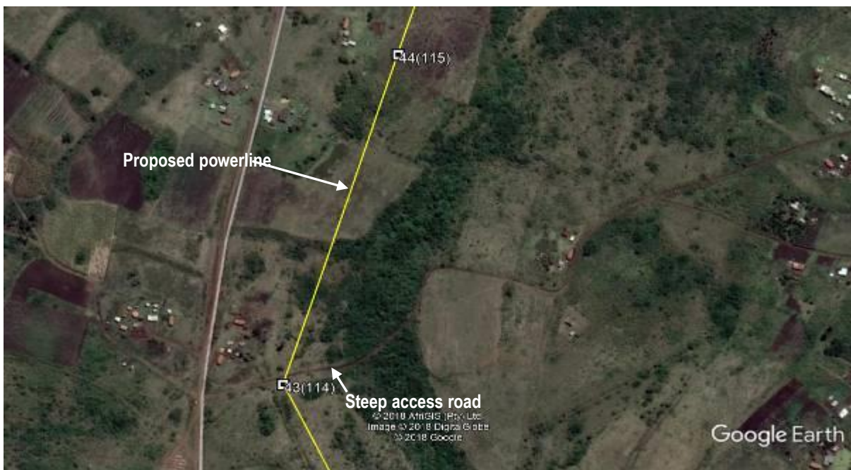
Fig. 31 Shows existing road with a steep slope and roads berms to be fitted along the road near tower 43(114) and trees within riparian area adjacent to a perennial stream 97
