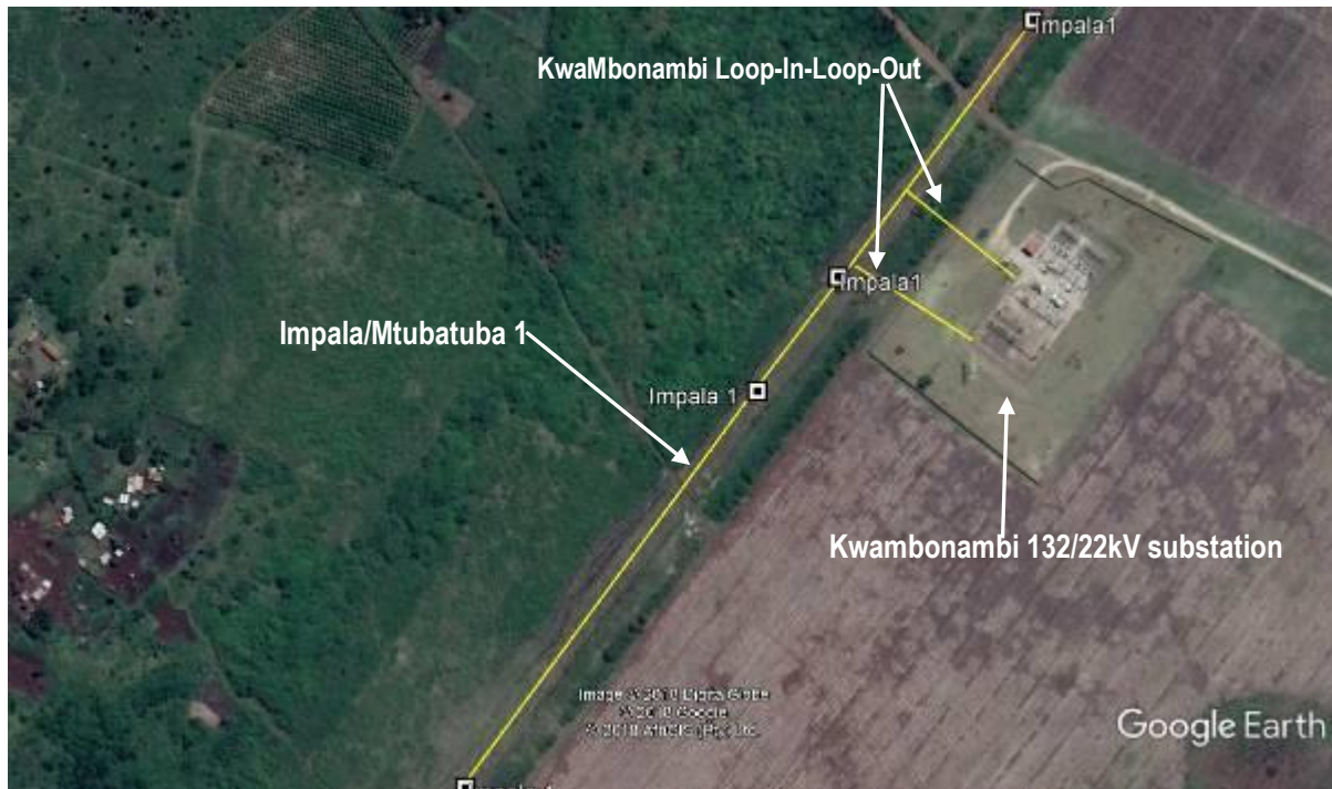
Fig. 52 Shows Impala-Mtubatuba 1 132kV powerline and KwaMbonambi Loop-In-Loop-Out Lines
