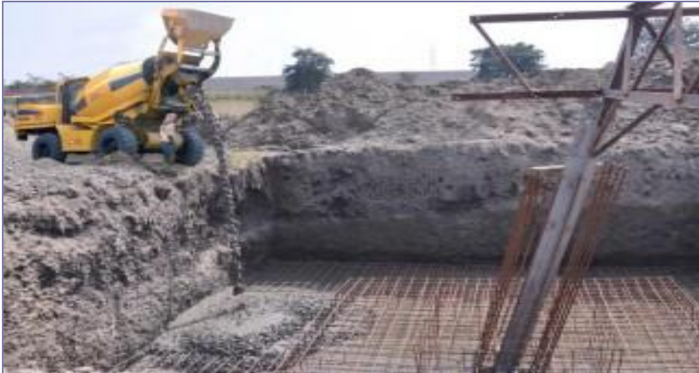
Fig 6 Pouring of cement into the tower foundation
