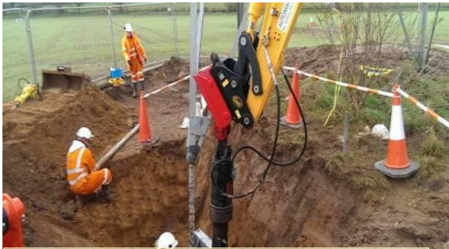
Fig 10. Shows the site area for the tower foundation
