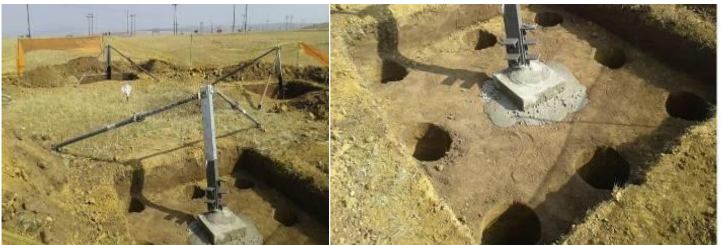
Fig 5 Clearance of ground cover and excavation of tow
